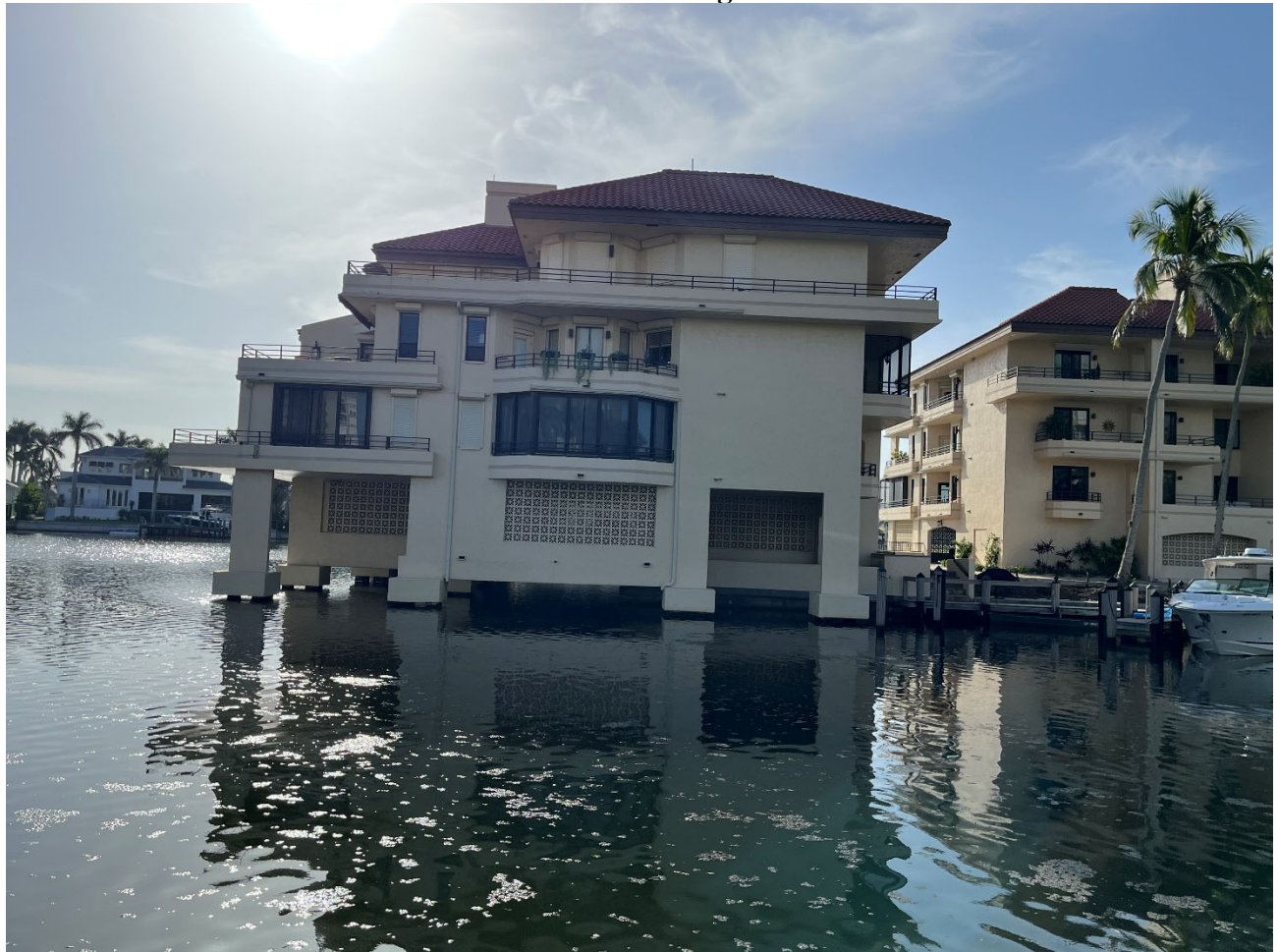
Front View of Building Six
