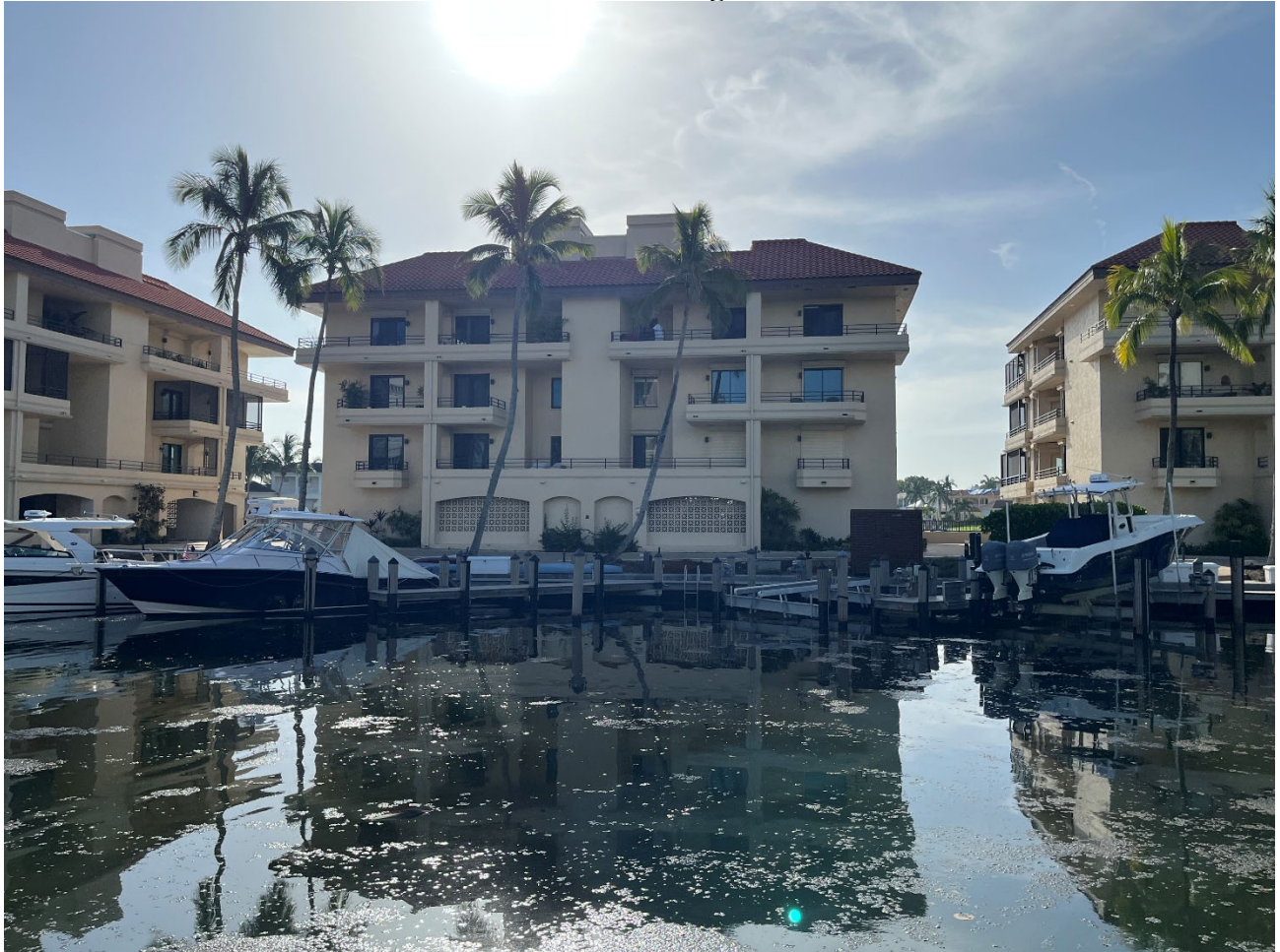
Front View of Building Five
