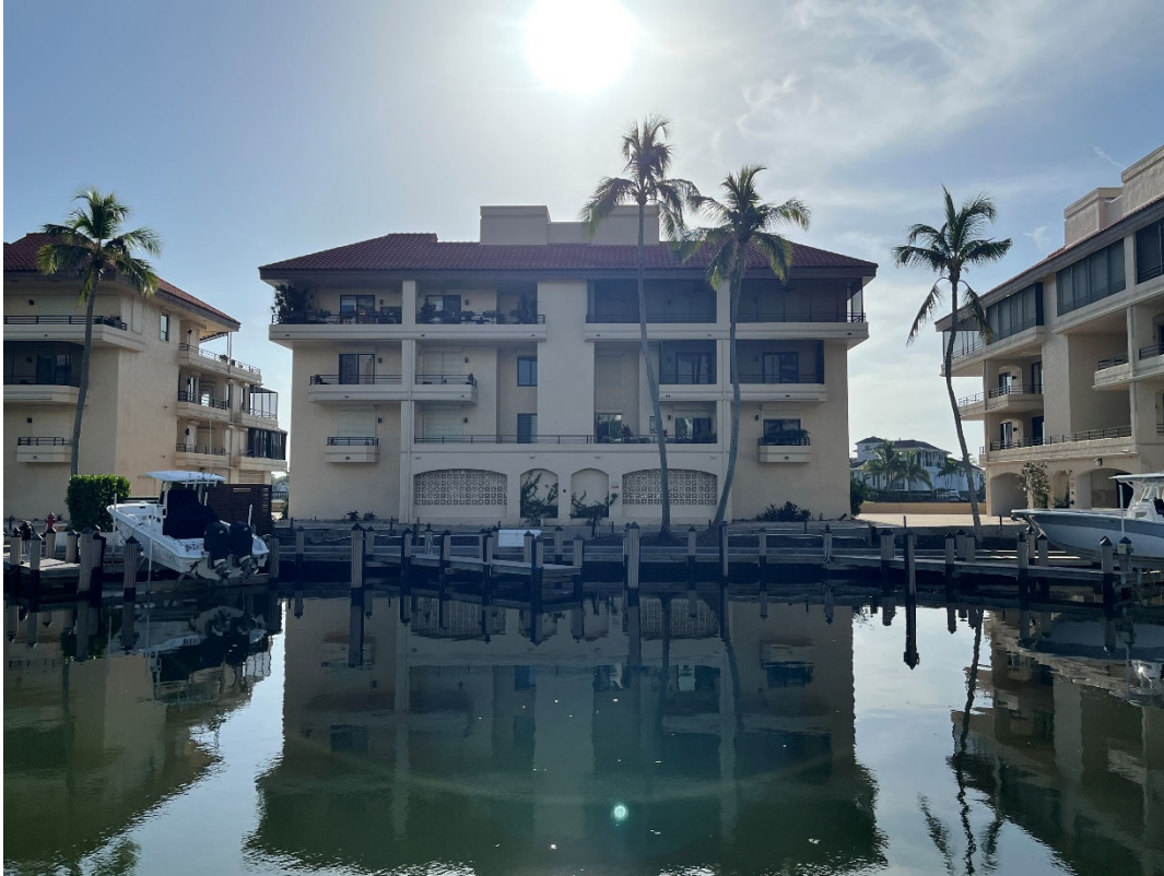
Front View of Building Two
