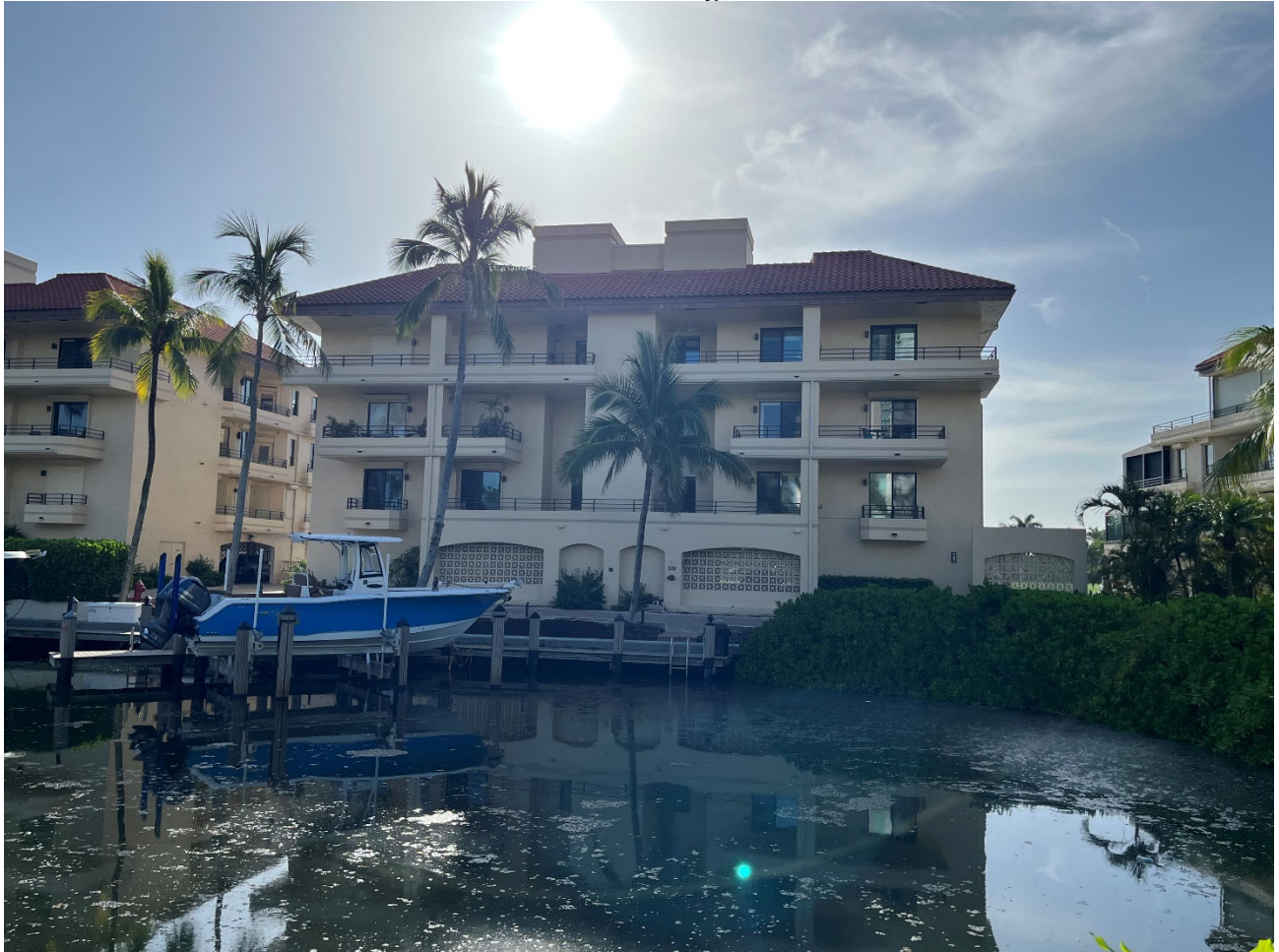
Front View of Building Four
